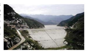
spillway tunnel, power stations at dam toe with a total reservoir storage of 28.1 million m<sup>3</sup>. The dam is a rockfill one with an asphalt inclined anti-seepage core covered by geo-synthetic membrane deck. The dam is of 85m high and 265m long with a crest width of 7.5m. The Reservoir is a standby reservoir for urban water supply.
